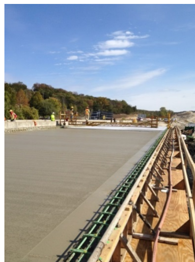
b) After Concrete Placement
