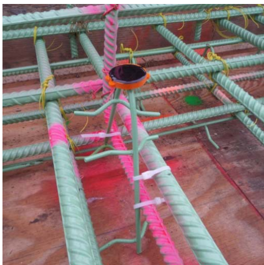
a) Before Concrete Placement
